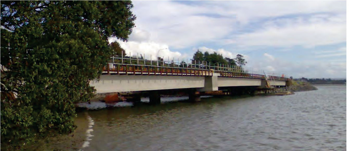
Figure 7: Example of a Super Tee bridge form
